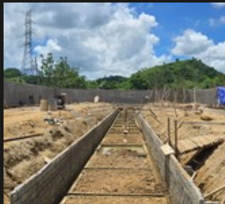
Pool foundation · longitudinal view with reinforcement
