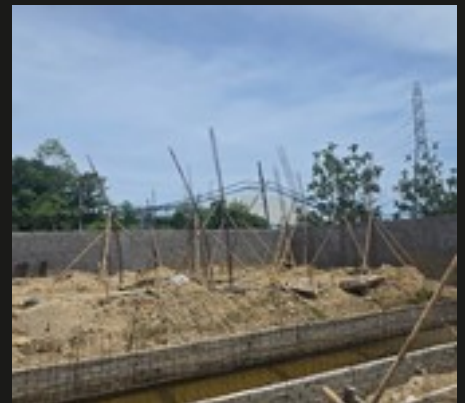
Reinforced columns with bamboo · site lateral view
