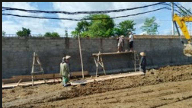
Perimeter wall · workers on bamboo scaffolding
