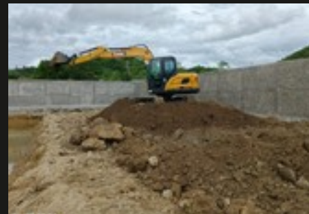
Earthworks · excavator in action
