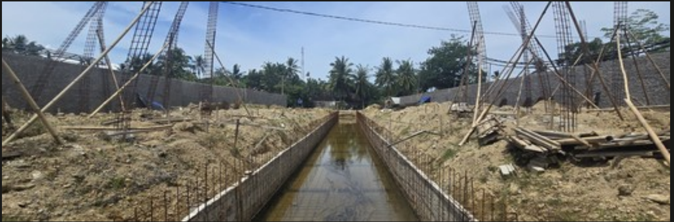
Panoramic view · column reinforcement and foundations · April 2026
