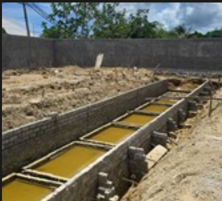
Linear pool · foundations and block walls
