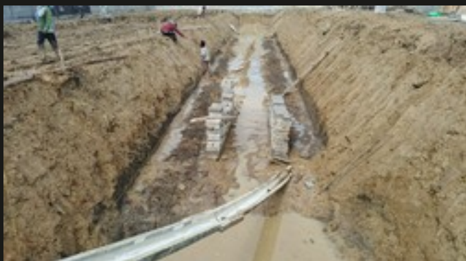
Pool foundation trench · base installation
