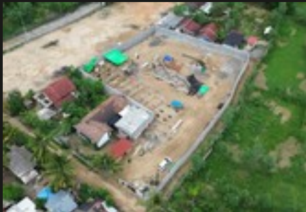
Aerial view · foundation works begin
