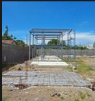
Steel structure · ground floor
