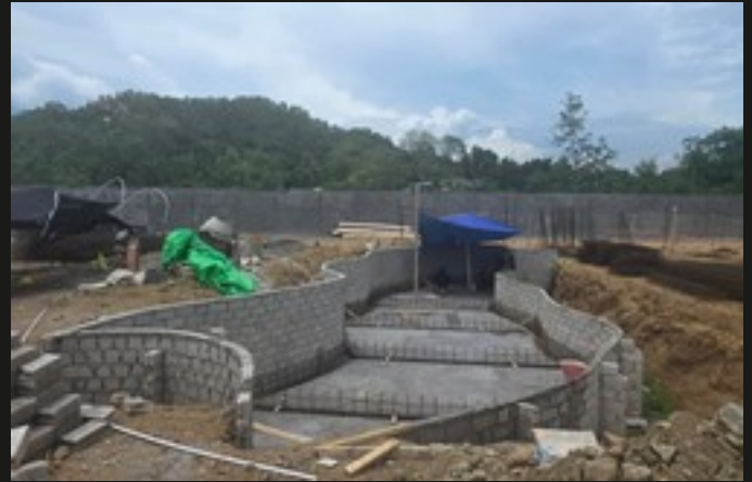
Aerial view · foundation progress
