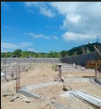
Foundations · column reinforcement
