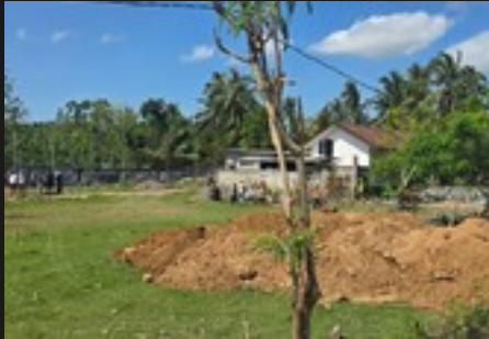
General site view · excavation begins
