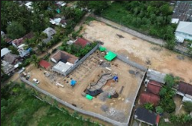
Pool construction · concrete and organic profiling
