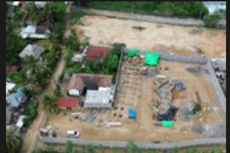
Front view · site progress
