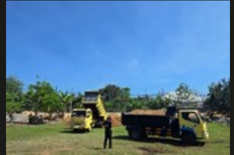
Soil import and surface levelling
